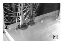
Wiring throughout the unit is neatly bundled and routed. Where wire harnesses go through the condenser bulkhead or blower deck, a molded wire harness assembly (19) provides an air-tight and water-tight seal, and provides strain relief. Care is also taken to tuck raw edges of insulation behind sheet metal to improve indoor air quality.
