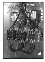
There is a blower contactor and compressor contactor for each compressor.
