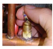
**A.** Remove the valve stem from the Schrader port mounted on the suction line.
