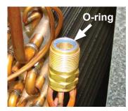
**III-2.** Replace the Teflon O-ring seal in place (located between the halves).
