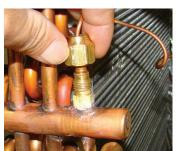
**B.** Screw flare nut on TXV equalization tube on to the Schrader valve stem.
