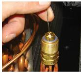
5. Pull the piston out using a small wire or pick. Verify the piston size (size is typically stamped on the body of the piston - Fig 7A-2). If a different piston size is required by the outdoor unit manufacturer, replace the piston using the small wire provided with the piston kit.
