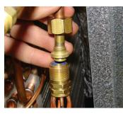
free of any residual pressure, disassemble the flowrator body completely using two wrenches. Take great care not to distort the feeder tubes. The wrench used to clasp the nut should be turned in counter-clockwise direction to unscrew the nut.
