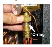
**III-5.** After ensuring that the Teflon O-ring seal is still in place inside the flowrator body, screw the female swivel nut onto the flowrator body.
